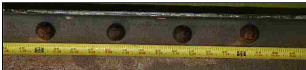
(a) West Channel Prior to Testing
