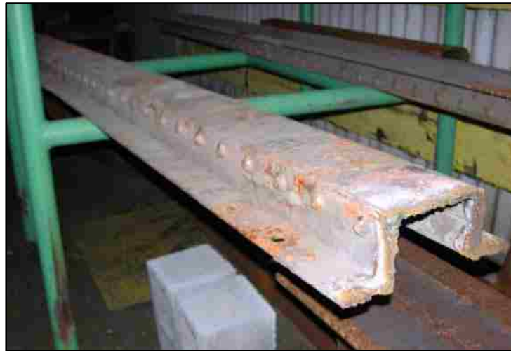
Figure 3.6 Original Guardrail Specimen
