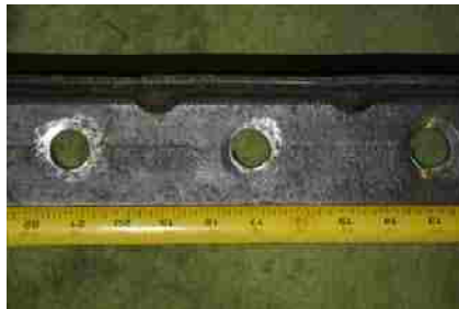
(c) West Angle After Testing
