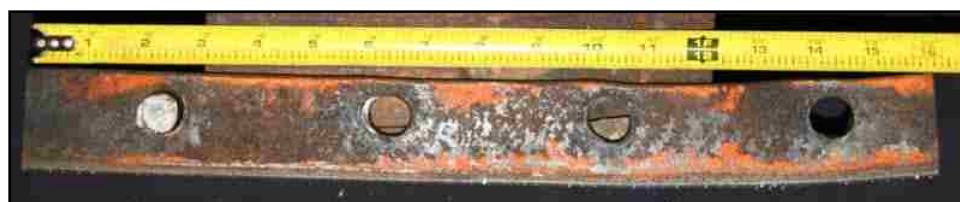
(a) East Channel Flange Faying Surface
